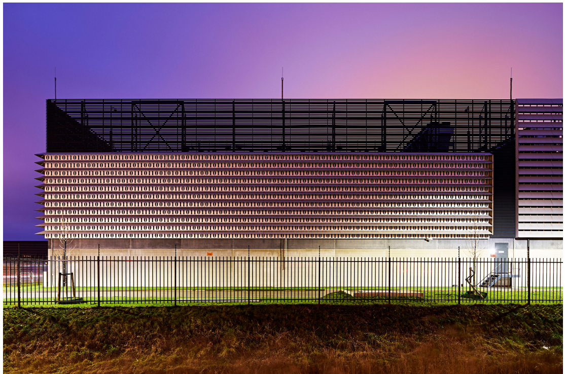
Interxion AM8 Datacenter, Rozenburg. – Photos by Niels Schrader and Roel Backaert
