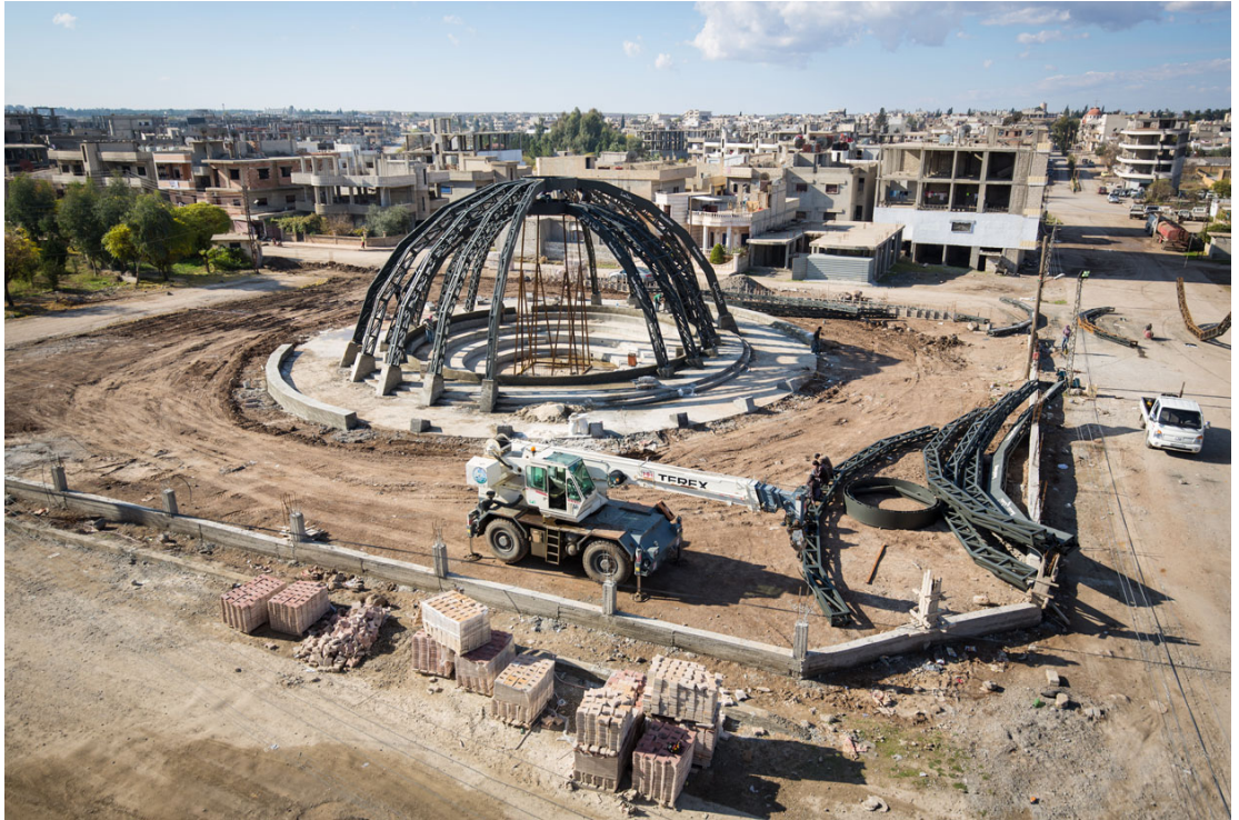
Construction of the new parliament and surrounding park in the city of Derik in the autonomous region of Rojava on 5 December 2015. Photo: Ruben Hamelink, New World Summit
