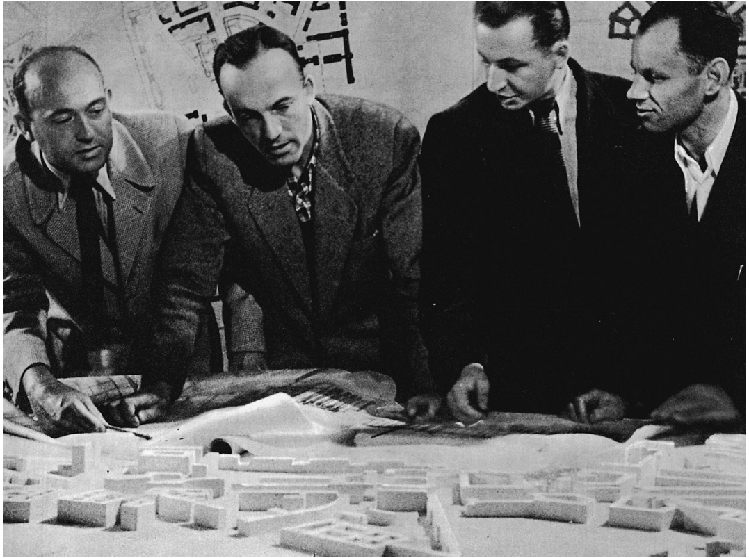
Meeting on the design and construction of the Marshalkovska Dzielnica Mieskaniova in Warsaw, early 1950s.
